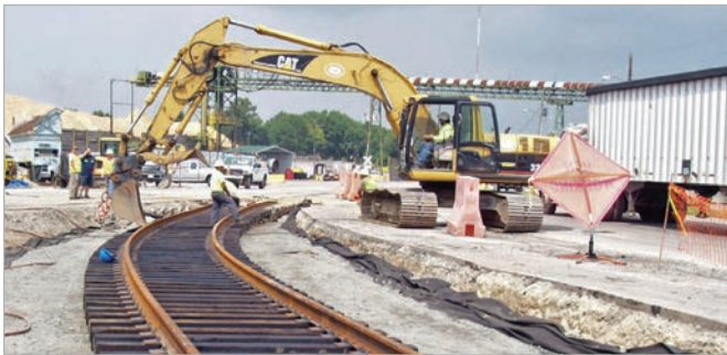
Track Improvements at Port of Wilmington
