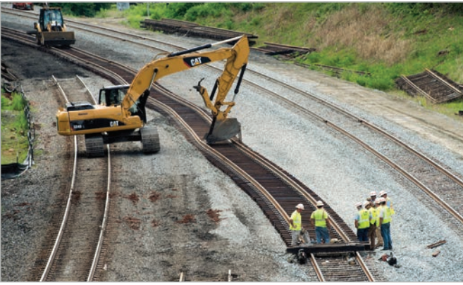
Previously passenger trains had to slow down to 45mph in Duke Curve. This curve realignment project allows passenger trains to travel up to 65 mph.
