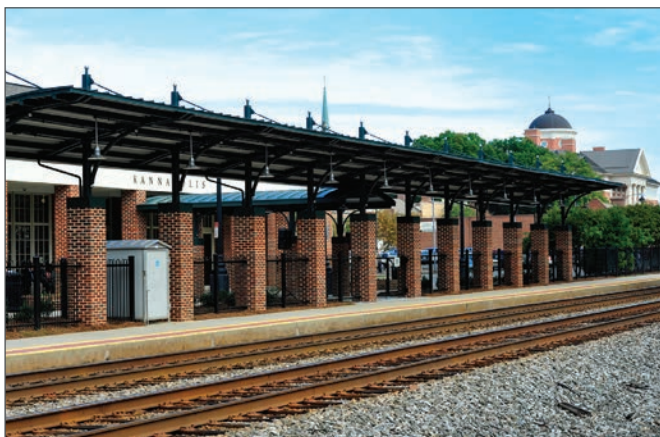
A new canopy was added to the Kannapolis Station with ARRA Funds
